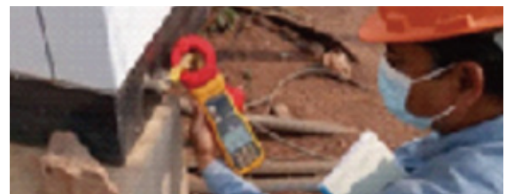
At our DRC mining site, we conducted inspections of flood and lightning protection systems in preparation for the rainy season.
