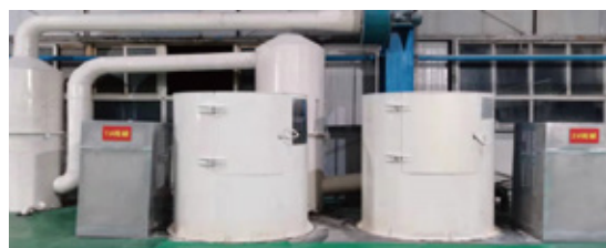
The No. 2 Tungsten Ore Processing Company in China uses a sprinkler system to reclaim dust from the flotation chemicals preparation process. This greatly reduces labor intensity and improves the work environment in the chemicals workshop, reducing exposure to occupational hazards.
