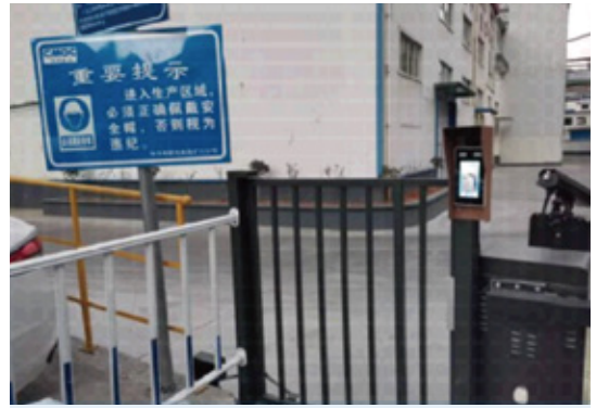
The entrance to our tungsten company has installed an automatic helmet detection system which prevents employees without a helmet from accessing the premises.
